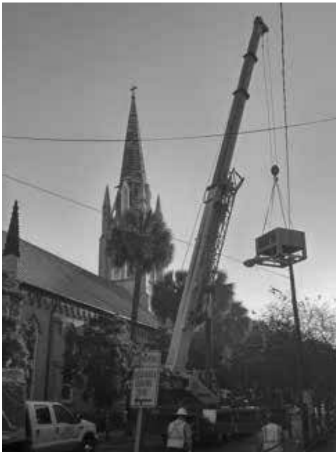
Left: Crane gingerly removing 1 of 3 “exhausted” heat/air units from west wing roof to make way for new, more efficient units. Just in time for summer!
